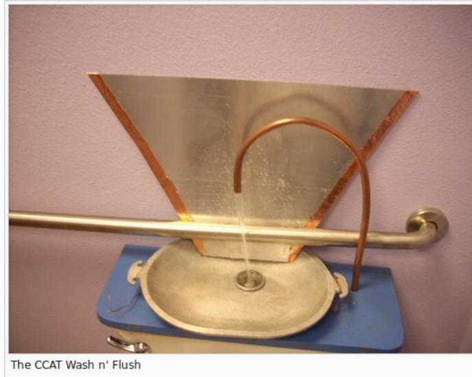
*A toilet modification that allows users to save water by utilizing the wastewater from handwashing to flush the toilet.*
